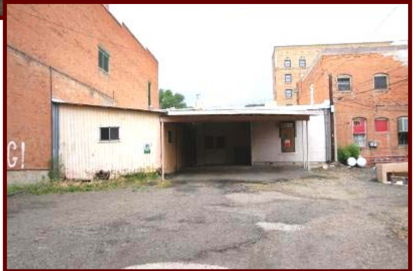
Carport in back
